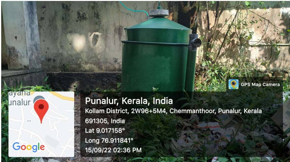
Biogas Plant setup near the College Canteen for local waste conversion.
